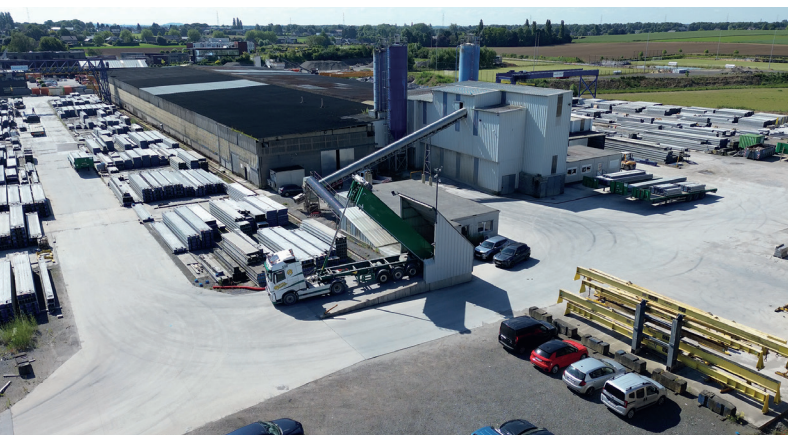
External view of the production plant of Ronveaux, located in Crisnée
