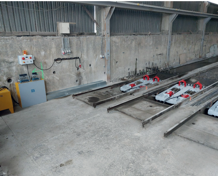
Fixed detensioning pump unit installed at the detensioning side
