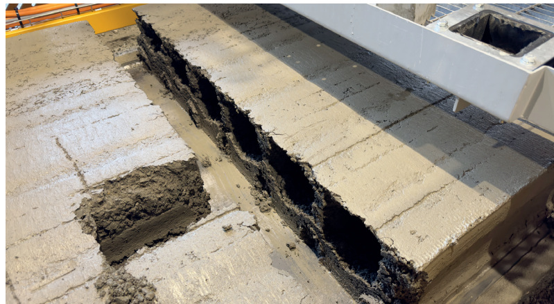
Quality of the fresh cutting with the guillotine system
