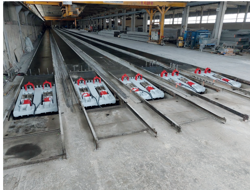
New reaction beams with detensioning
