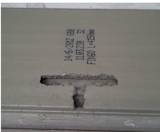
Typical work openings on fresh concrete
